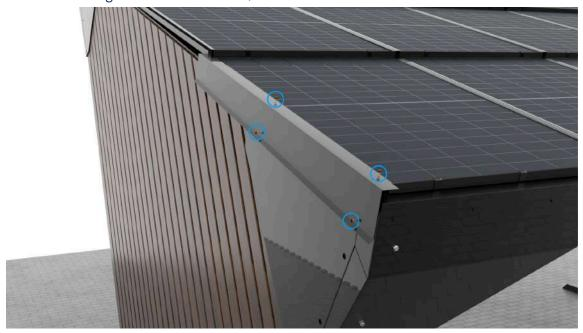
• Connect the side flashing starting from the bottom corner. The edges of the upper side flashings must overlap the lower ones.
