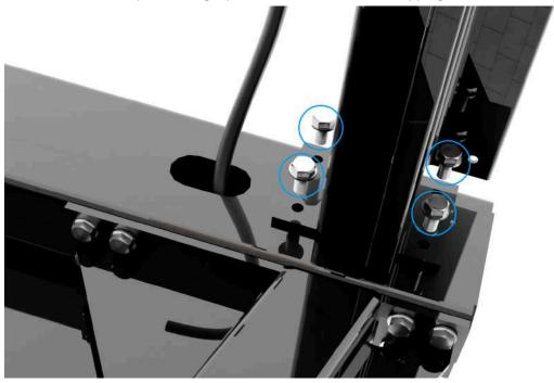
• Secure the eave purlin diagonal brace using 12 pcs of SFS TDBL-13.4 self-tapping bolts per brace.
