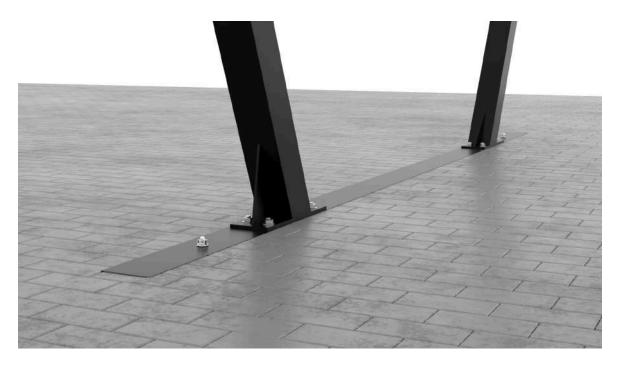
• The ground rises and sags during the winter period due to freezing the anchor connections should be checked and tightened annually!
